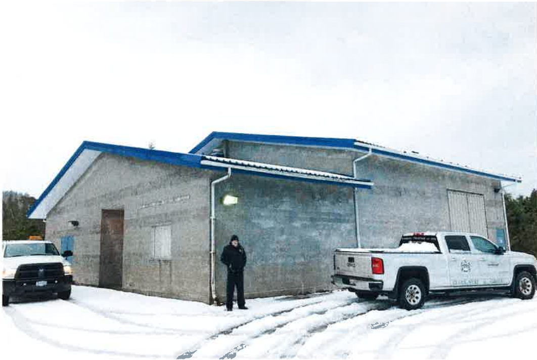
Figure1: Port Edward Water Treatment Plant Main Building
