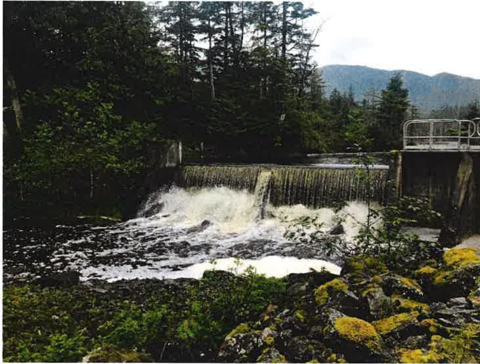
Figure 2: Alwyn Lake Dam and reservoir
